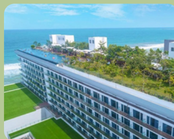
(a) Green roof
